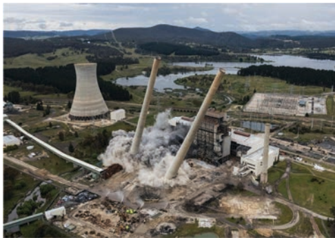
Rethink: Phased and controlled demolition
