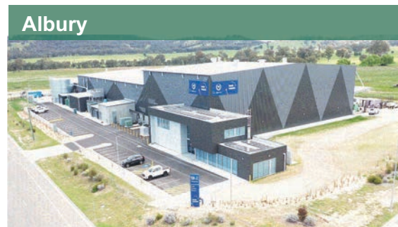
2021: Construction of a new 28ktpa PET recycling facility in Albury
