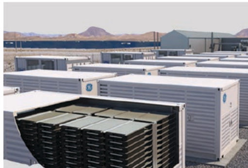
Regenerate: Development application lodged for the Wallerawang 9 Battery
