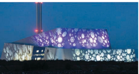
Covanta, Dublin, energy-from-waste
